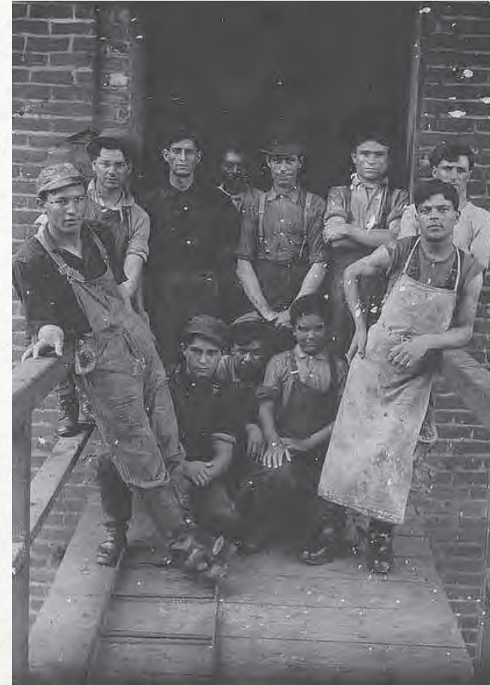
The Swift Bldg was first constructed in 1909 and was used as a meat packing and distribution refinery for Swift & Company.
