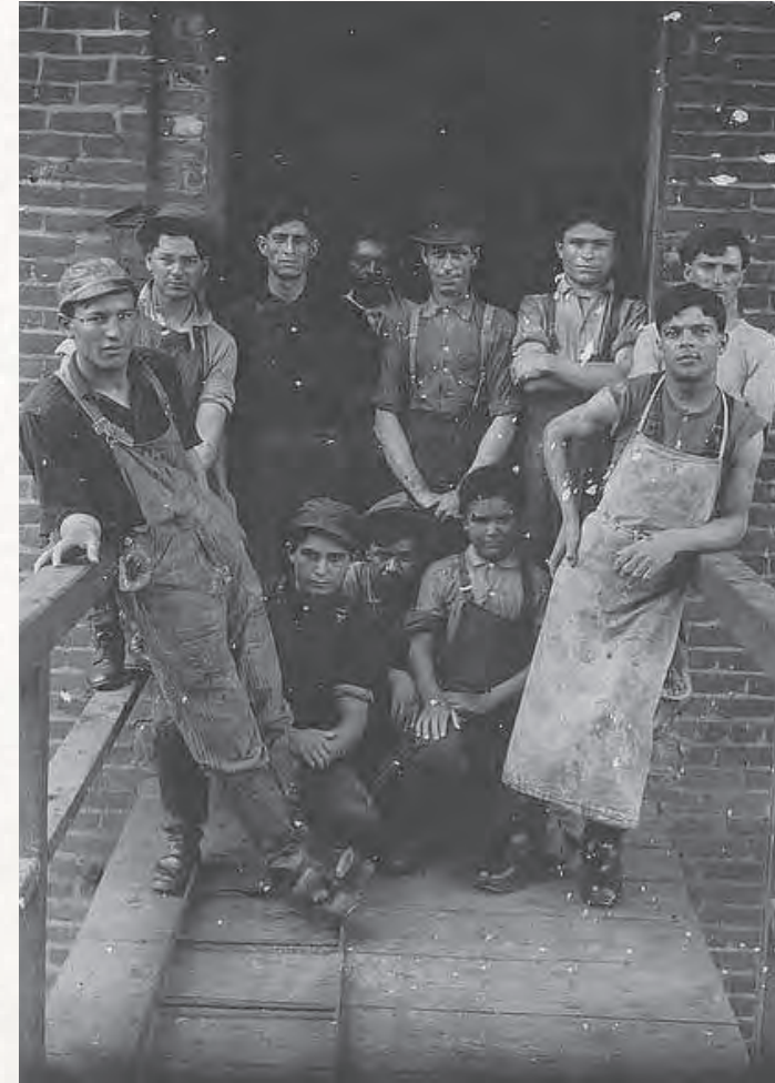
The Swift Bldg was first constructed in 1909 and was used as a meat packing and distribution refinery for Swift & Company.
